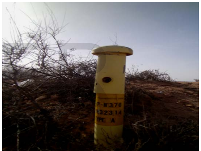
Figure 2.8 -Test post number 370 at 323.14 km from Brega city
