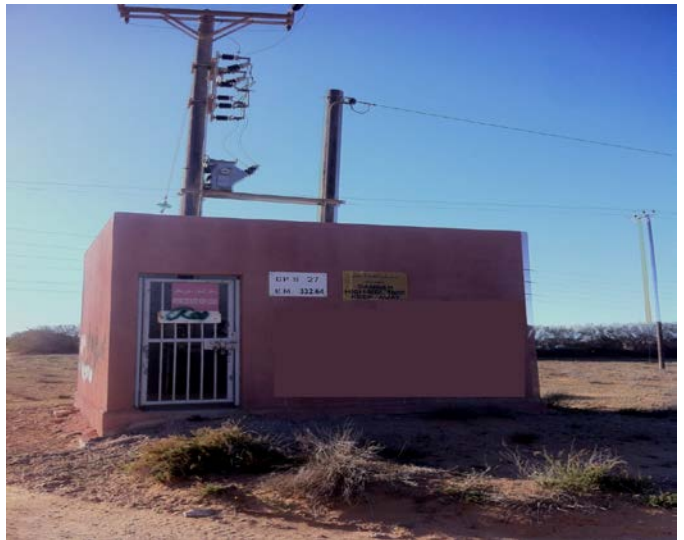
Figure 2.7- Station number 27 at 332.64 km from Brega city.
